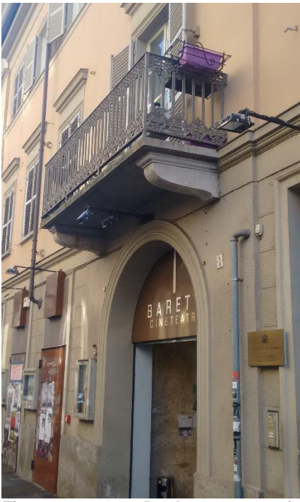
Figure 76 Deployment of SLM000349, via Baretta 4, temporary
