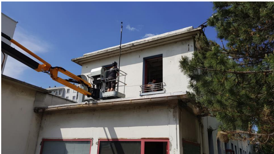
Figure 16 Sound Level Meter at artist's lodge rooftop
