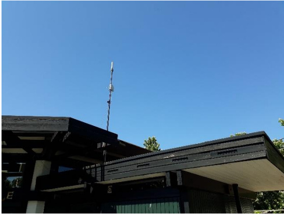
Figure 4 Master unit at command center
