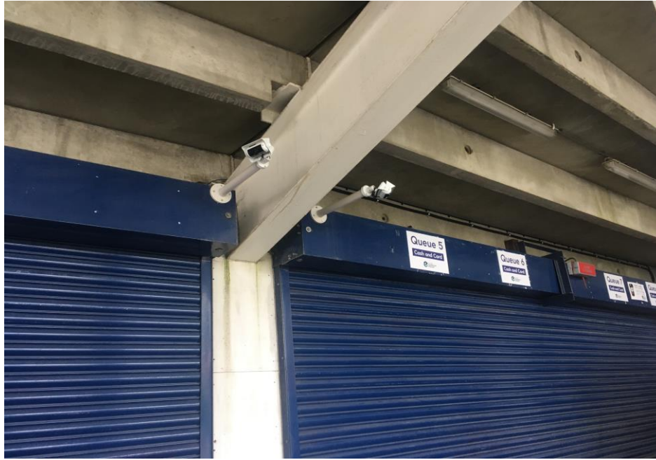
Figure 43 Time of Flight cameras installed over the bar area to observe queues
