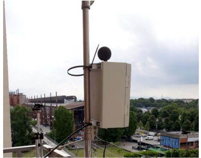
Figure 28 B&K SLM on a building in Via Orvieto
