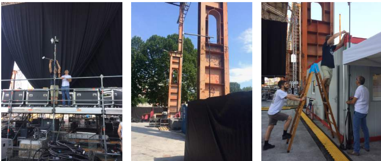
Figure 35: Setting up the anchors in the test area
