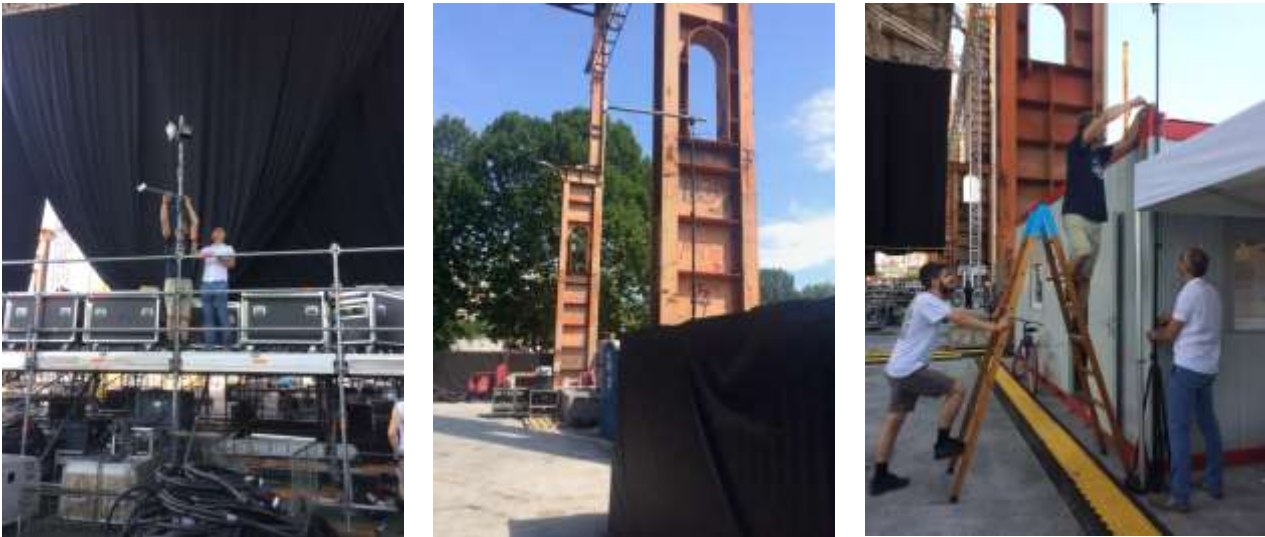
Figure 26: Setting up the anchors in the test area
